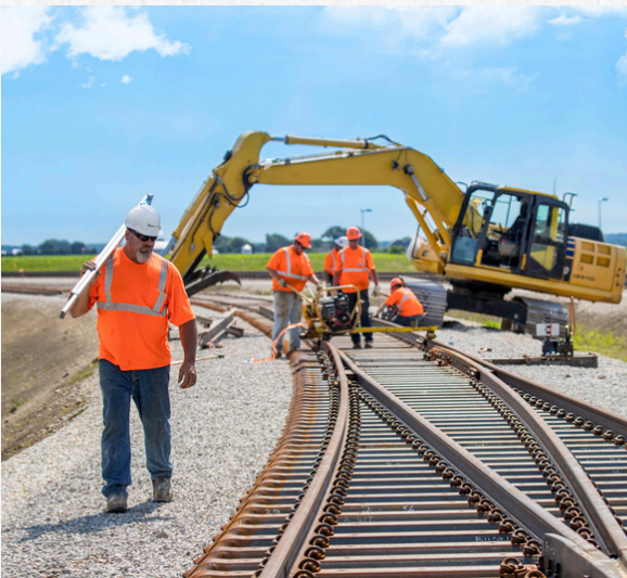
RAILWAY TRACK CONSTRUCTION
